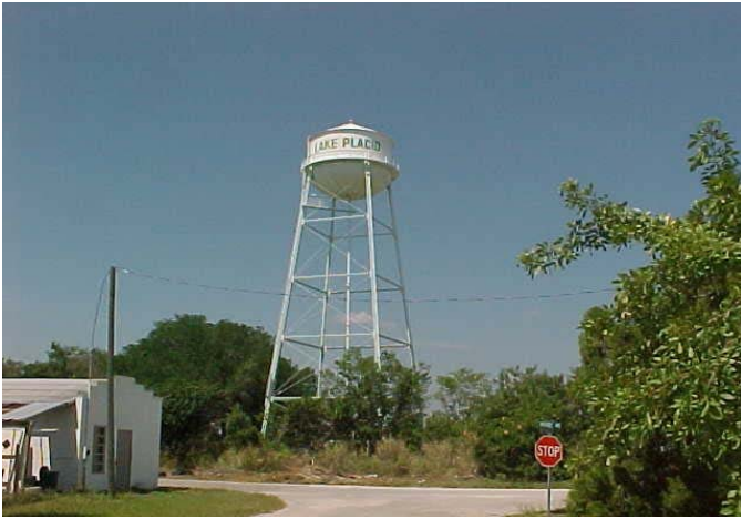
DEWEY ELEVATED WATER TANK
